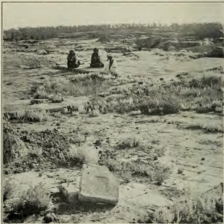
FIG. 10.—Floor of Nebuchadnezzar's Temple as it Appears To-day, Showing Blocks Joined by Means of Asphalt.
